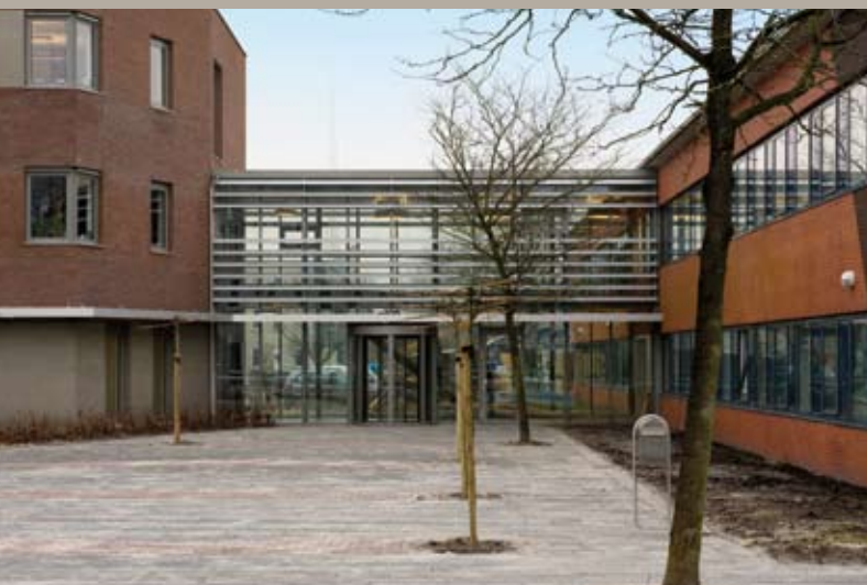
Kantoor Promens Care Assen ↑
